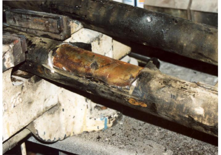
2. The beam with the knuckle removed
