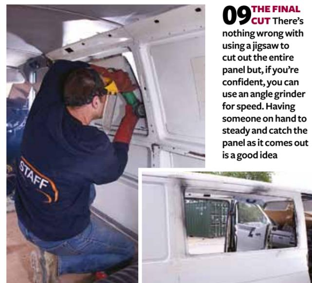
**09 THE FINAL CUT** There's nothing wrong with using a jigsaw to cut out the entire panel but, if you're confident, you can use an angle grinder for speed. Having someone on hand to steady and catch the panel as it comes out is a good idea
