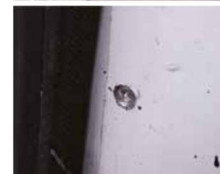
**05 DE-BURR** The drill got rid of most of the welds, but there will always be bits remaining that will hold the panel in place. We ran along these areas with a cutting wheel on an angle grinder so there were no 'hang-ups' when we came to remove it
